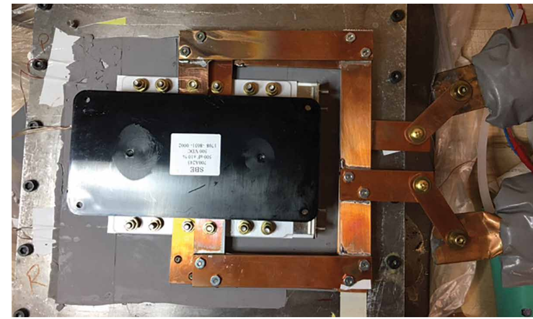
Figure 3. SBE 700A243 500μF 500V integrated capacitor/bus installed on cooling plate and connected to ripple current source for temperature rise testing.
