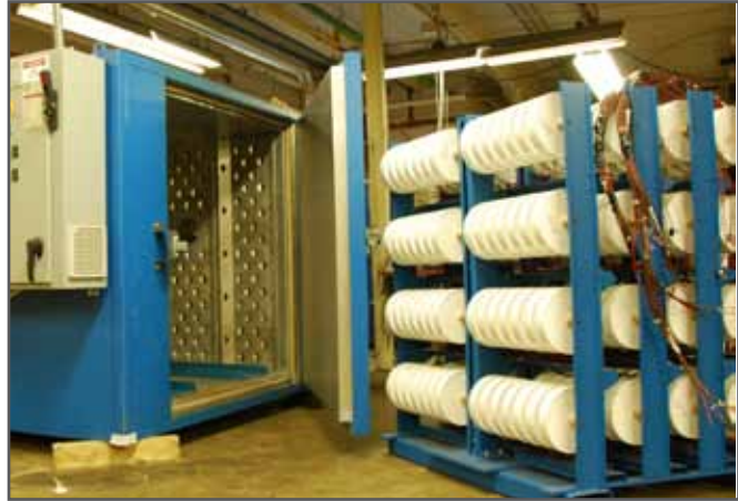
Figure 1: A population of 224 Power Ring capacitors installed on a support rack prior to loading into the thermal chamber.
